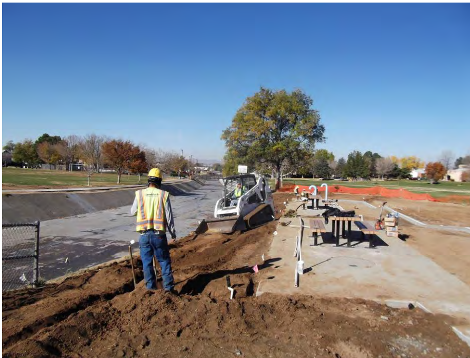
RMCI backfilling for Land Tek at Montgomery Park.
