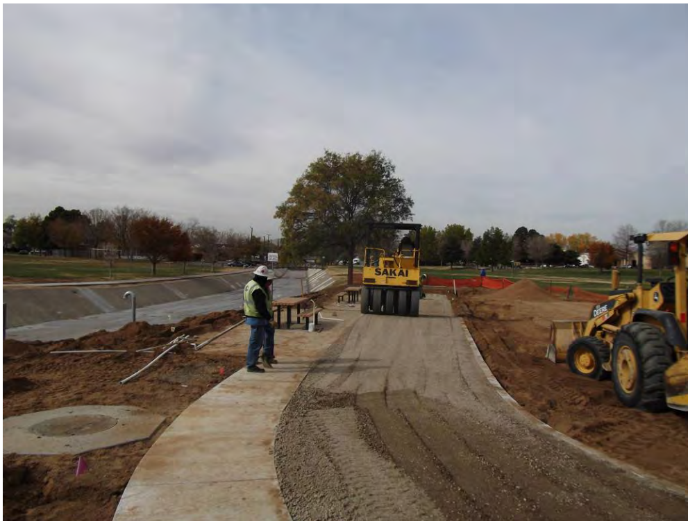
AAI rolling base course at roadway in Montgomery Park
