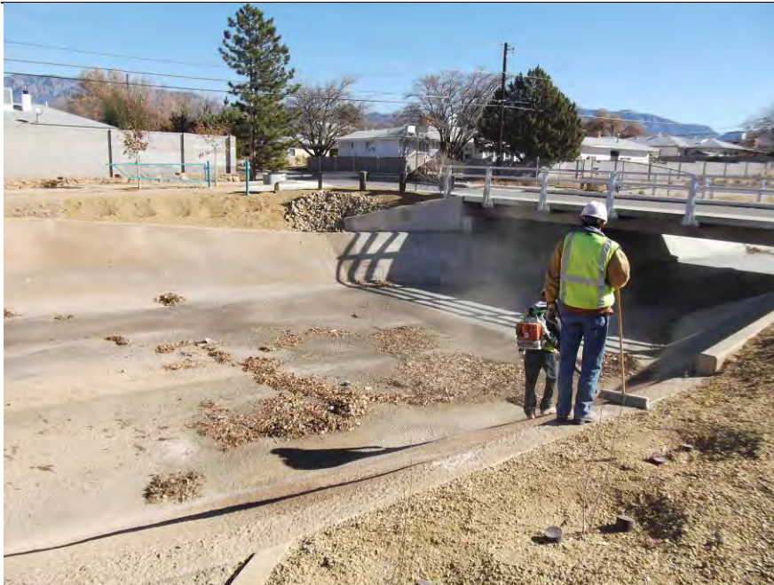
RMCI cleaning the channel.
