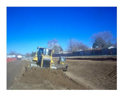
Dozer is processing the 1 ft subgrade prep. The loader with a laborer is picking up the concrete debris as it rolls out.
