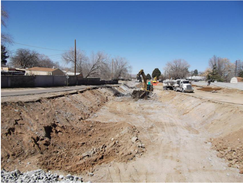
Guzman removing channel lining West of San Pedro.
