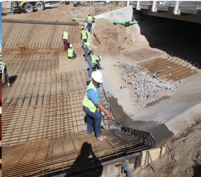
Contractor placing lithium on existing concrete. This is the first application.
