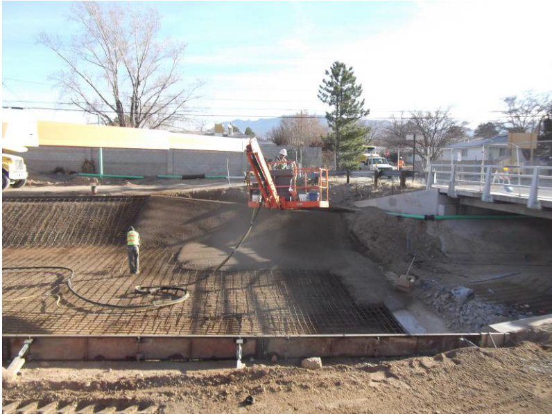
Superior tying into the existing channel.
