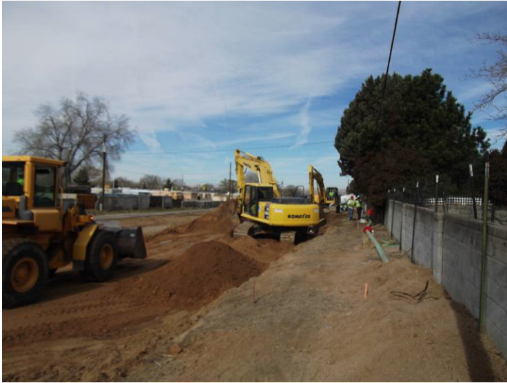
RMCI placing the 24" PVC at about Sta. 12+50
