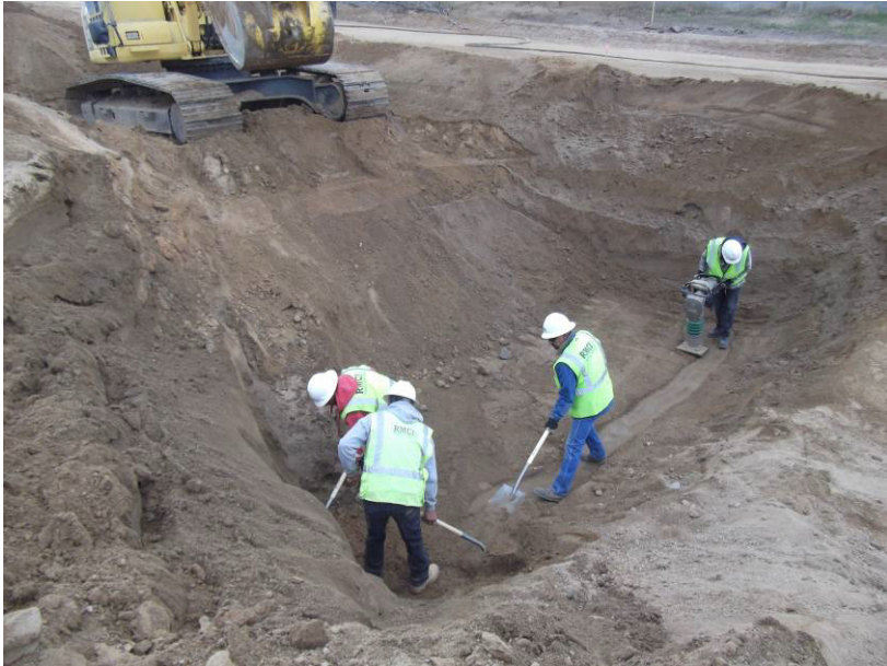
RMCI digging out material for cattle guard. Crews processed the dirt for 1' subgrade prep.
