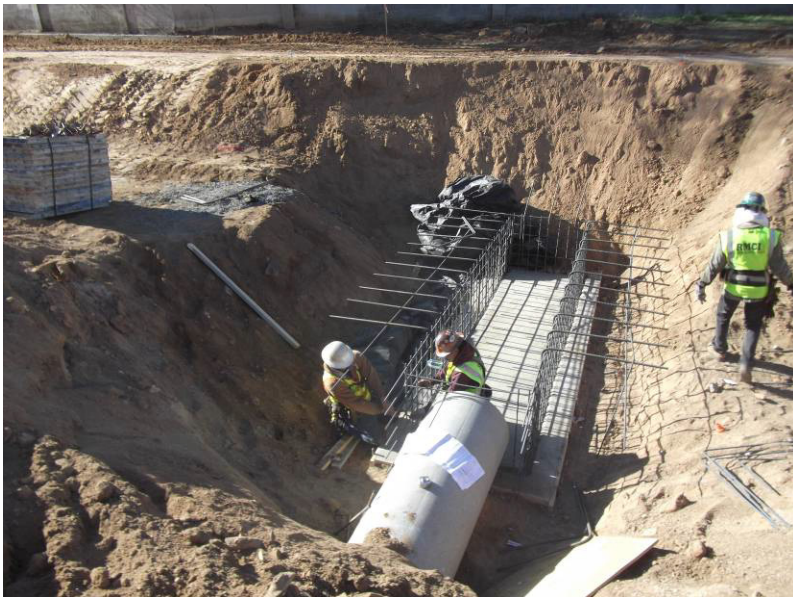
PRS placing rebar at cattle guard.
