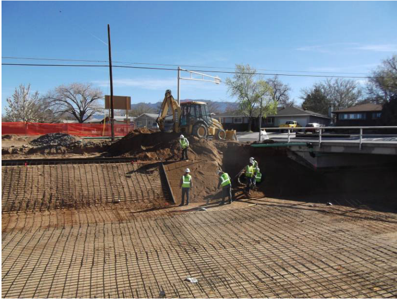
RMCI began working on 18" RCP Pipe Penetration
