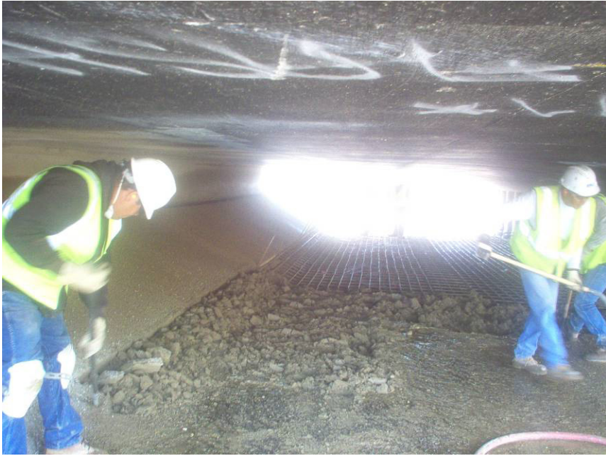
Contractor removing shotcrete that was damaged by storm waters.
