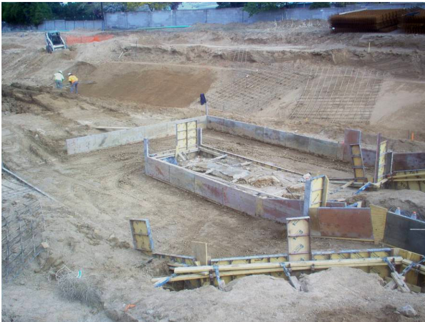
Contractor removed silts and rebar mats from the WQS.
