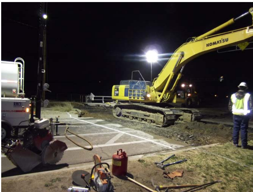
RMCI removing asphalt and trenching for the 24" DI. Sat. night
