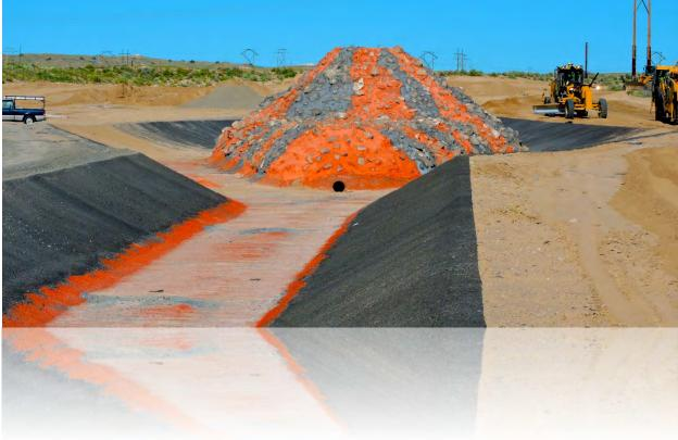
Modeled at the UNM Hydraulics Lab and then implemented near I-40 and 98th Street, this volcano 'erupts' with stormwater to increase the oxygen content before water flows to the river
