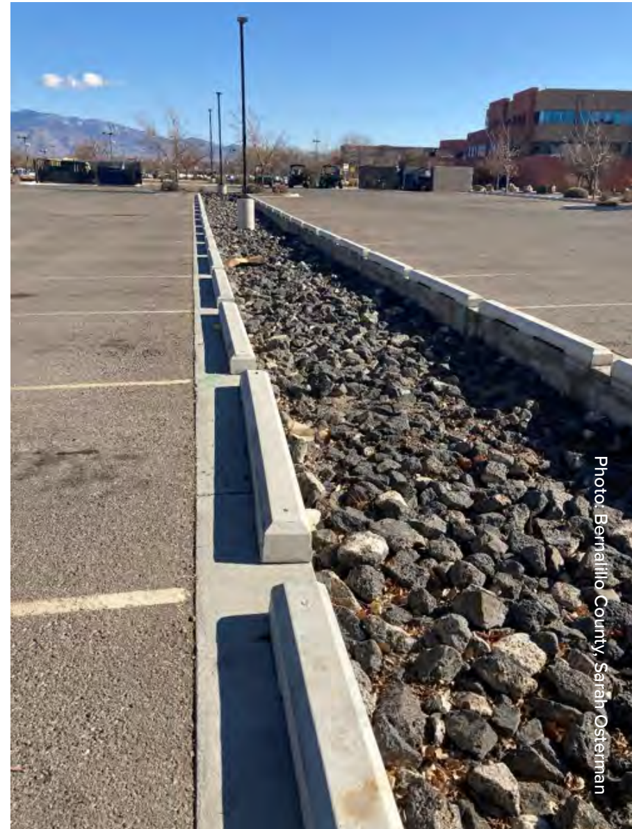
Infiltration trench in parking lot
