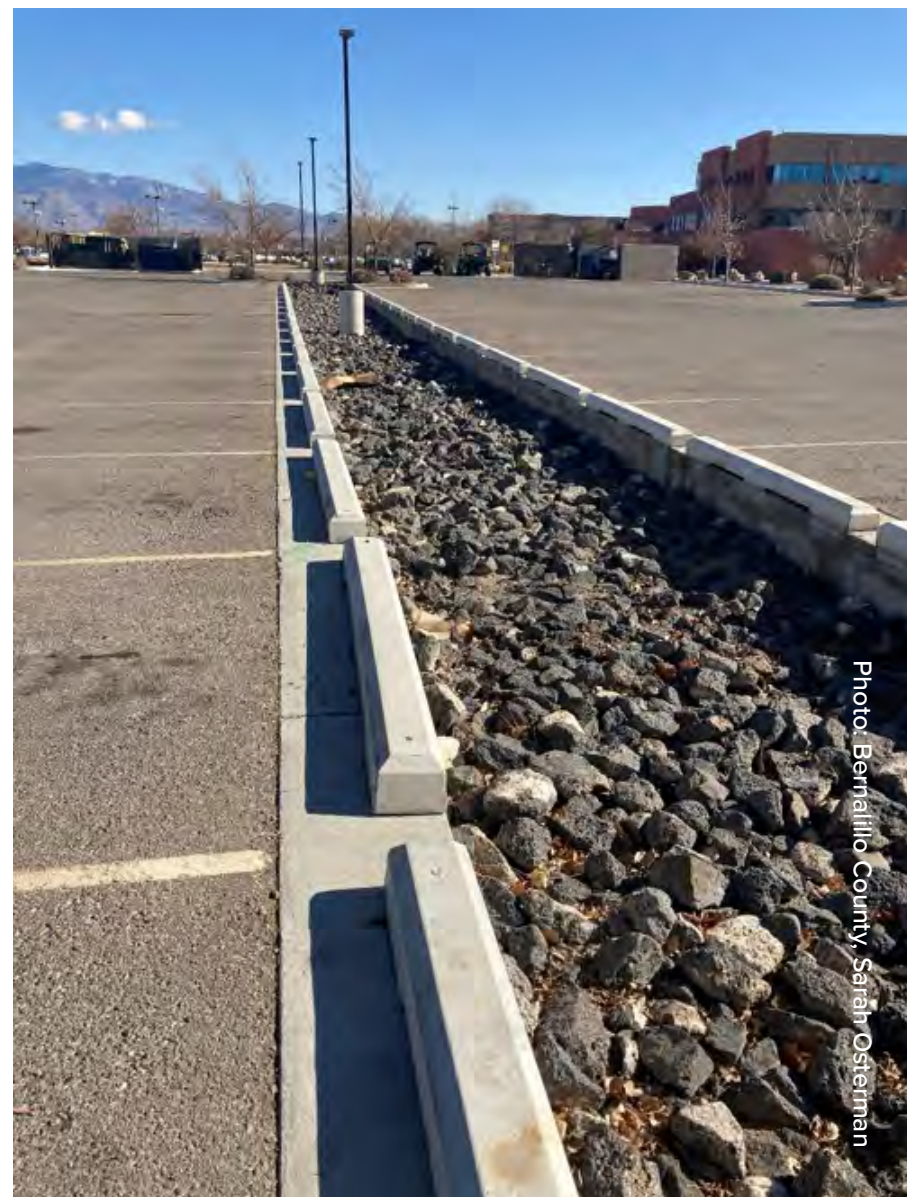
Infiltration trench in parking lot
