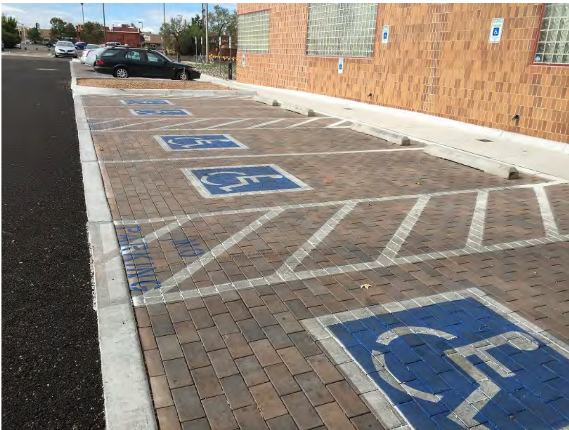
Wheelchair accessible permeable pavement
