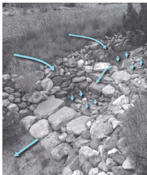
Left: Stormwater harvesting basin at CNM
