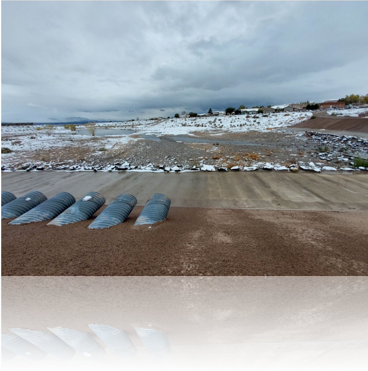
Black Arroyo Dam
